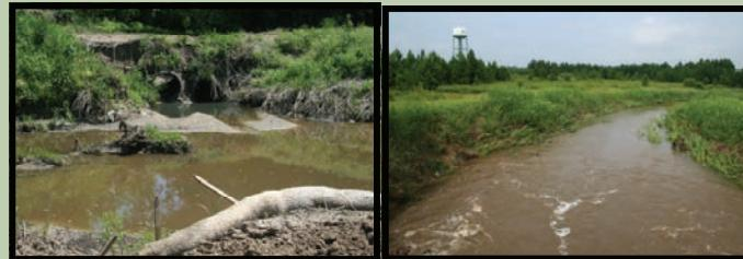
The Corps of Engineers excavated an 8-mi canal through Crabtree Swamp in 1965-66 for drainage. This narrow channel causes water to flow very rapidly.
