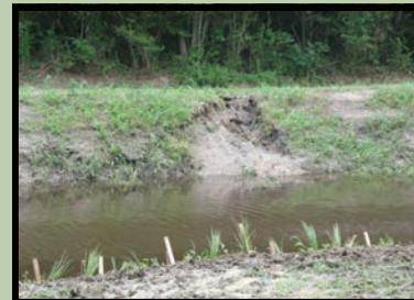
This has lead to serious erosion of the canal banks, as well as other water quality challenges.
