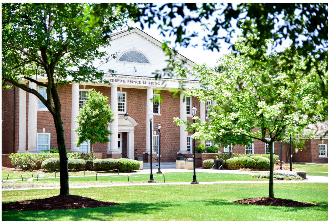
Eldred E. Prince Building at Coastal Carolina University
