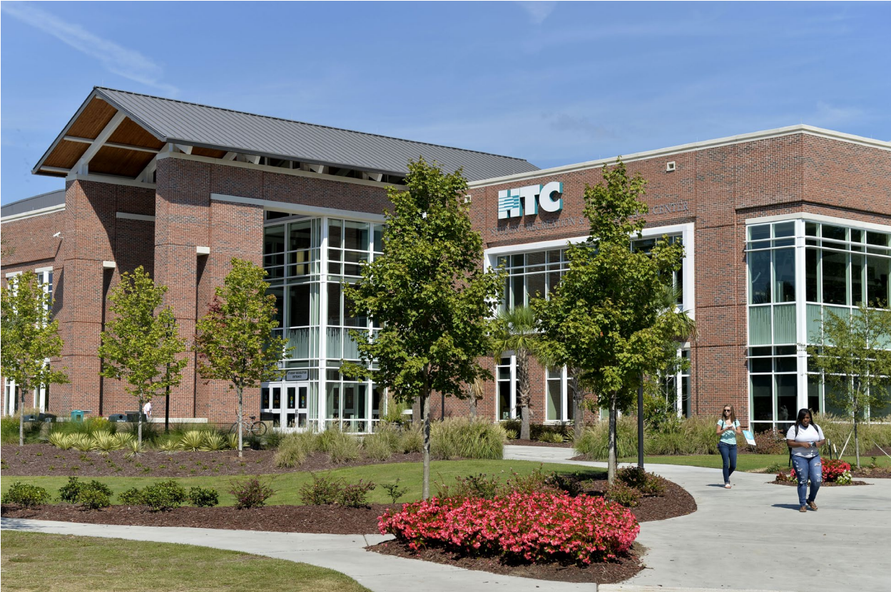
HTC building at Coastal Carolina University
