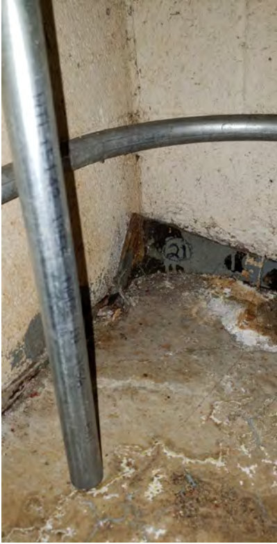
Base molding located in the front left mechanical room
