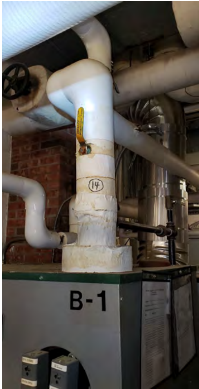
Insulation covering on approximately 4-inch soft/fiberglass insulated pipe connected to B-1 equipment located in the front left mechanical room
