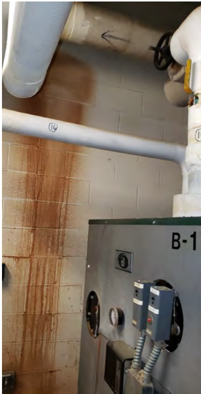
Insulation covering on approximately 4-inch soft/fiberglass insulated pipe connected to B-1 equipment located in the front left mechanical room
