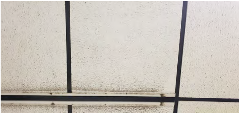
Ceiling tiles - located throughout
