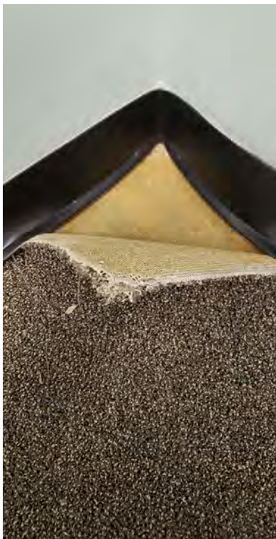
Mastic associated with multicolored carpet located throughout the 2nd floor
