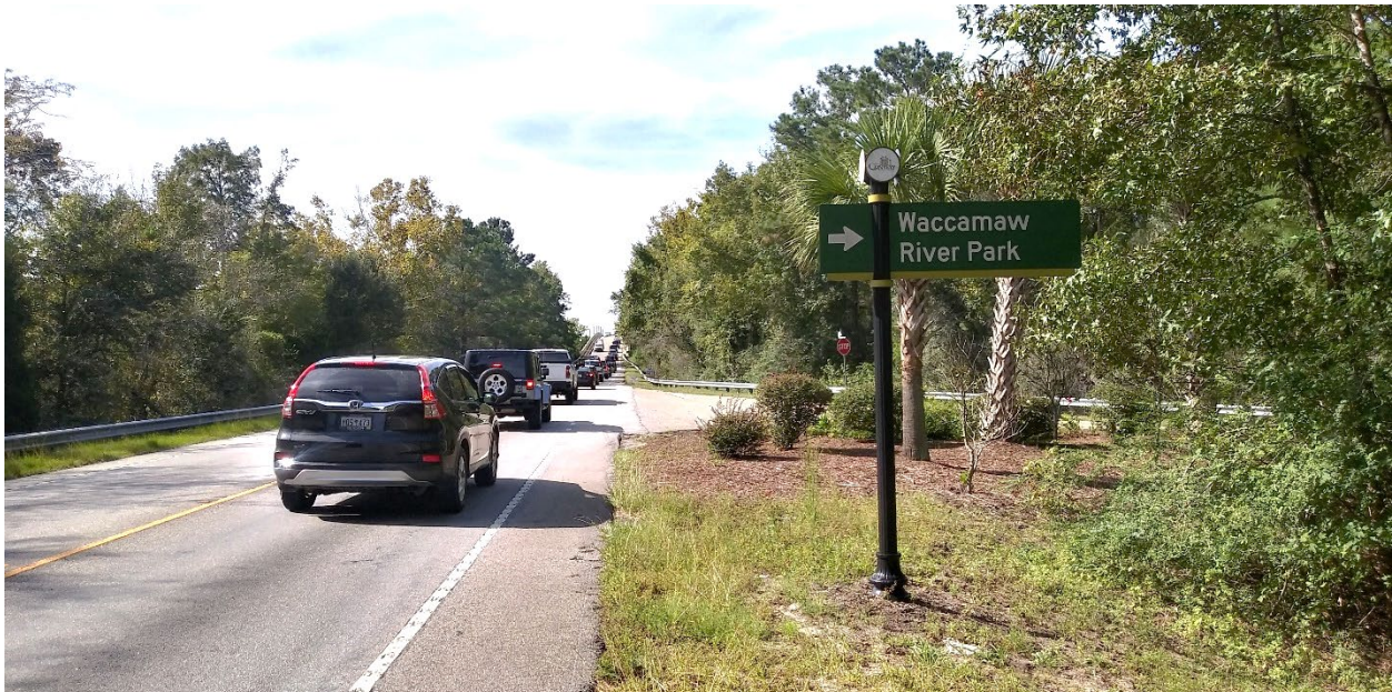
Figure 10. Northbound traffic on 501 Business entering downtown Conway, with the Main St. Memorial Bridge in the distance and the entrance to Depot Road and the Waccamaw River Park to the right. Also note the rumble strips lining the unofficial bike lane. Photo: Sara Rich.
