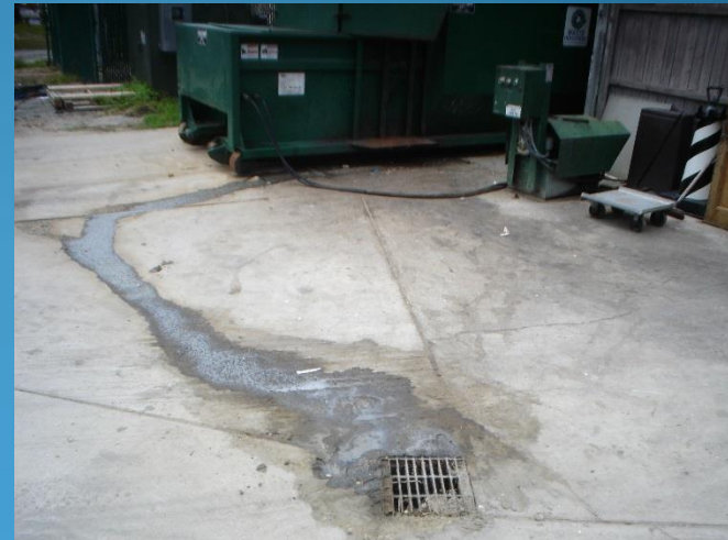
Dumpster Leak
