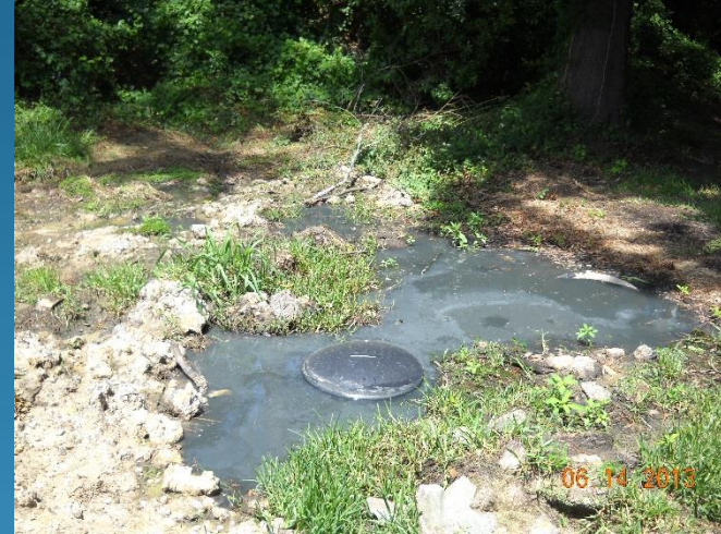
Failing Septic
